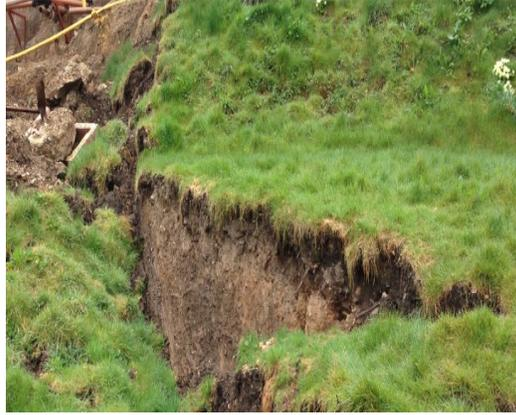
Bad practice in earthworks which may cause erosion during construction
